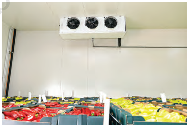
Fig. 12.12. Cold storage facility for vegetables
